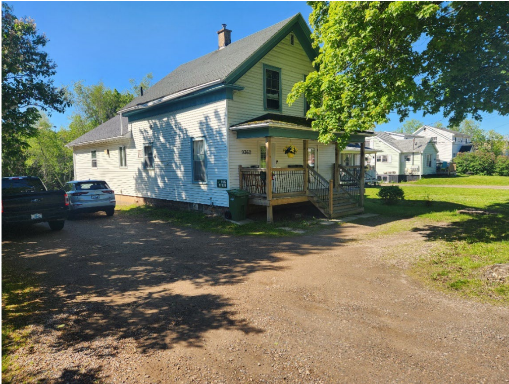
Subject property with the four-unit dwelling and neighbouring property to the west
